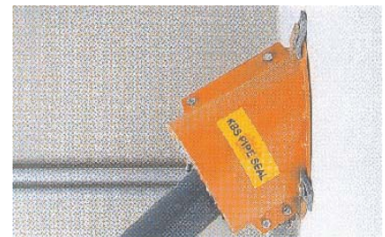
KBS Pipe Seal M-DI
