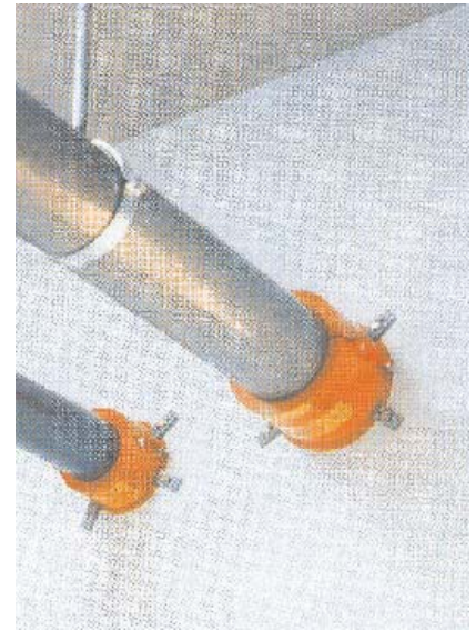
KBS Pipe Seal S and M
