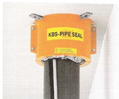
Pneumatic tube with cables in KBS Pipe Seal M
